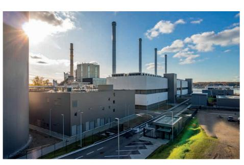
20 Jenbacher J920 FleXtra gas engines make up the heart of the coastal power plant, generating 190 megawatts of electrical power for the German city of Kiel. "Photo Copyright -Stadtwerke Kiel"
