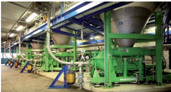
Solids pumps KOS 1050 in sewage works ProReno (Basel, Switzerland)
