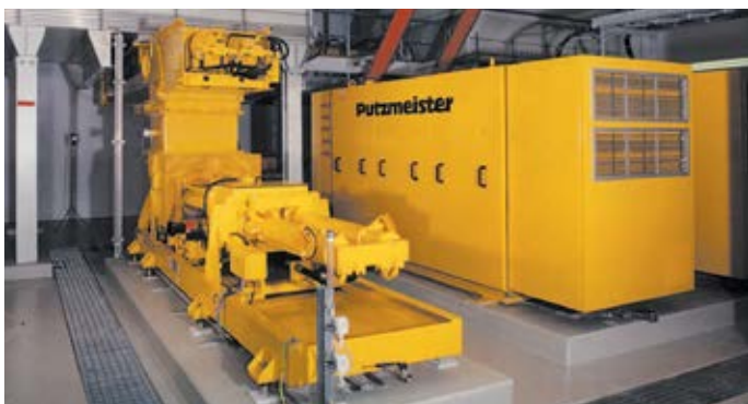
Co-incineration of sewage sludge in the coal-fuelled power station Zolling (Germany): solids pump KOS 2180
