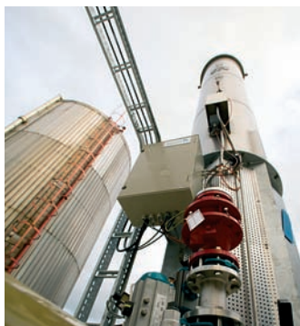
Biogas burner for safe combustion of an-digestion gas.
